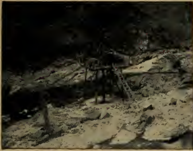
Well No. 1 Showing Pumping Pier Above Flood Water.
